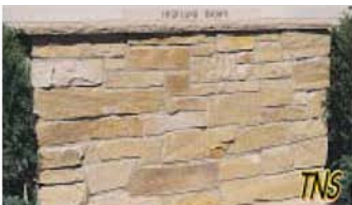
Highland Brown Ashlar – Random ashlar pattern offering a blend of light and dark browns and tan colors.
